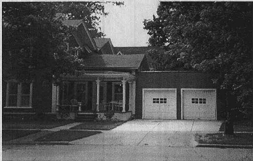
Two garage doors are preferable to one large door. Historic details were most likely destroyed by attaching this garage to the house. Detached garages are preferred.
