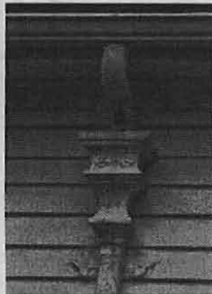
Gutters, downspouts, and mounting brackets may be features to be preserved.
