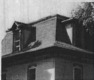
The dormers and roof slope are characteristics of the Italianate style of this house, and should be preserved. Such features should not be added to historic homes that never had them.
