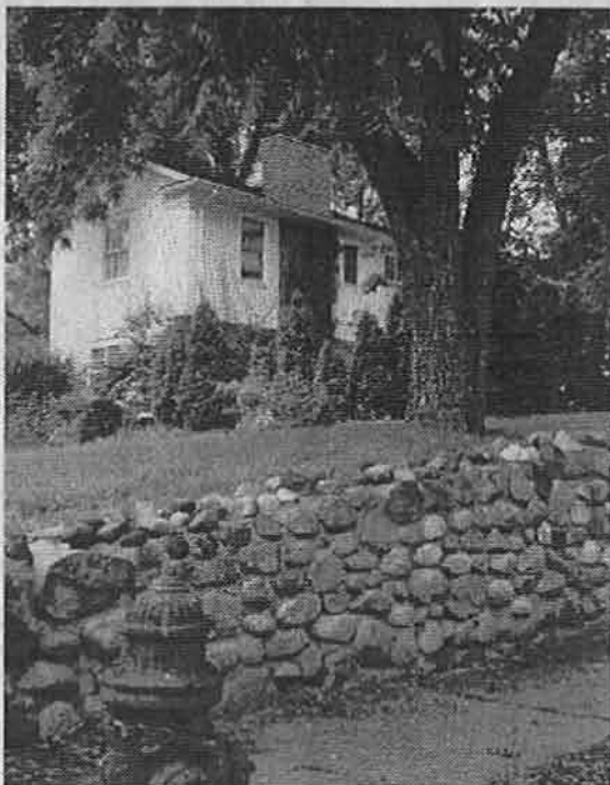
Historically appropriate retaining wall.
