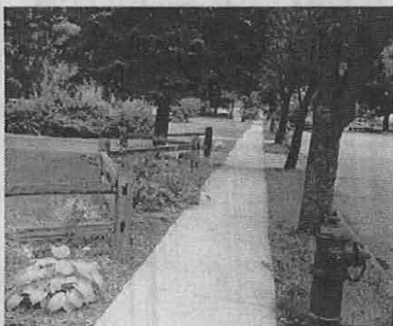
This fence meets the Standards for height, but the split rail detailing is more appropriate to a rural setting. It may not meet zoning requirements.
