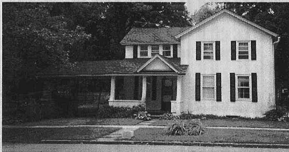
Damage to historic materials is less with a carport addition. In this case the roof should not be continuous with the porch roof, a prominent feature of the front of the house.
