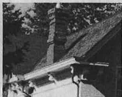
The chimney, fascia, and carved brackets are roof features to be preserved.
