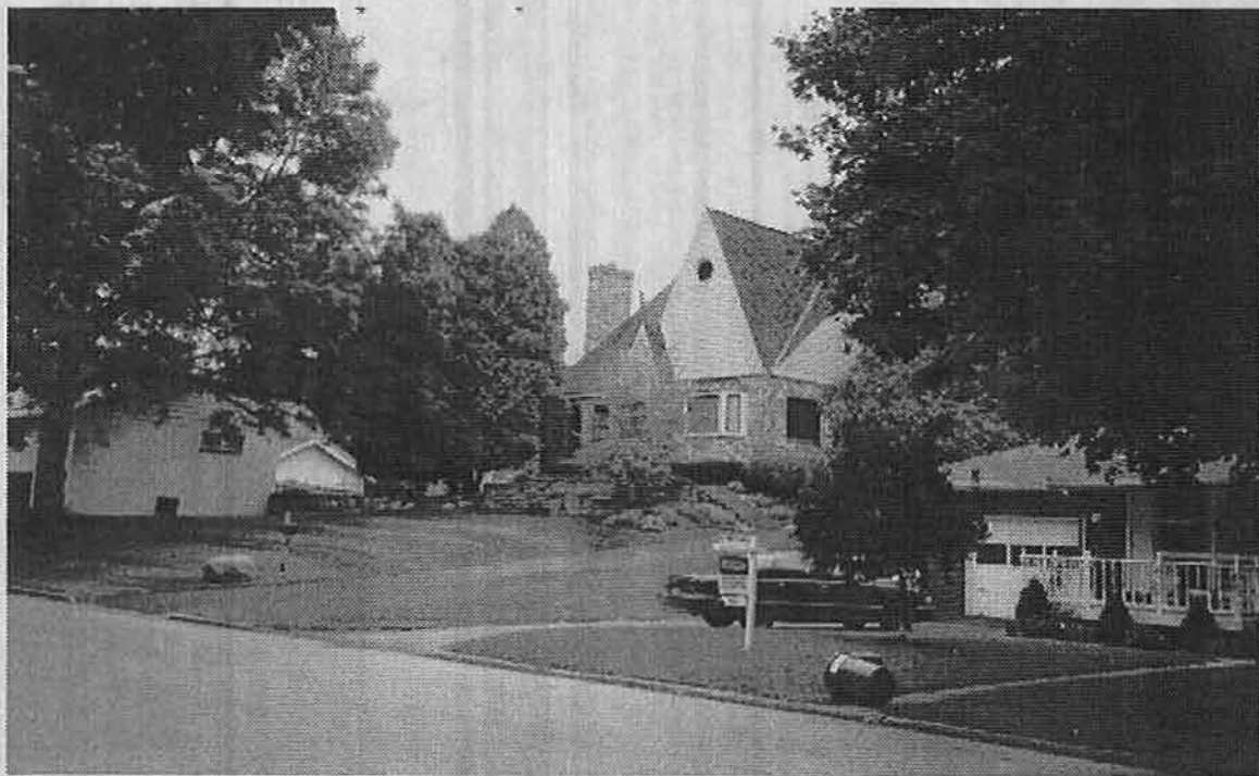
The house in the middle is set back much further than its neighbors. Although probably in keeping with zoning, it does not follow Historic District Standards for compatibility.
